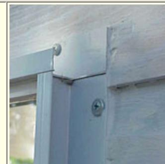
I also caulked all the gaps where the scalloped part of the siding met the window flange. This will deter leaks and discourage bugs from nesting in there.
