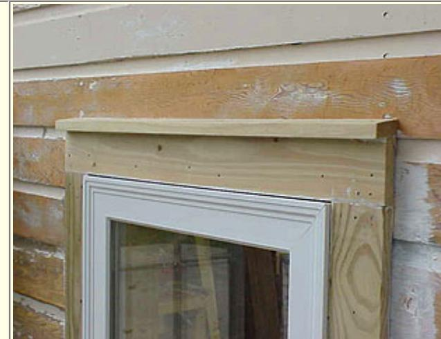
The completed casing, ready for priming and painting.
