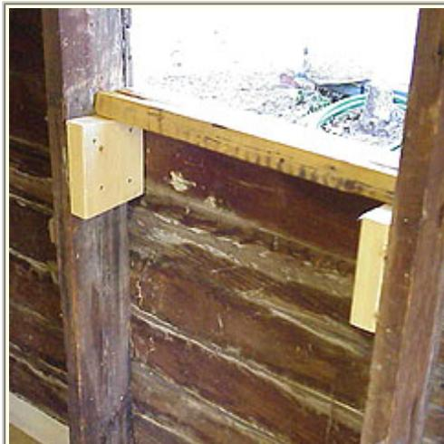
After the sill was stripped and sanded, I installed two angled blocks for the sill to rest on. I was careful to make sure that the sill would end up level, because the window will rest on this sill.
