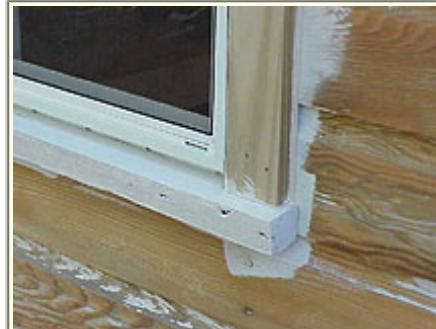
The bottom end of the side casings were cut at a 10 degree angle to match the window sill.
