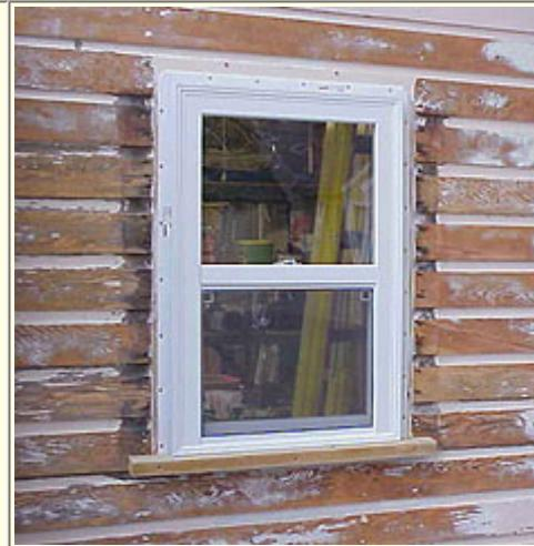
The window with the faker-sill attached at the bottom.
